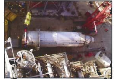
Getting ready to lift reactor from ground transport vehicle.
